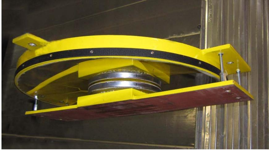
Figure 4. A typical standard pendulum isolator bearing, viewed from below.
