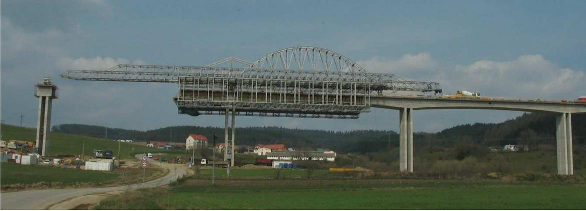
Figure 1 - MSS for the construction of a 70m span bridge in Slovakia
