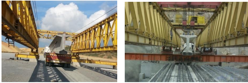
Figures 6, 7: Views from the installation activities performed in V7.
