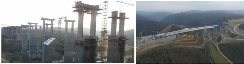
Figures 8, 9: Works performed in V6 Viaduct by ILM.
