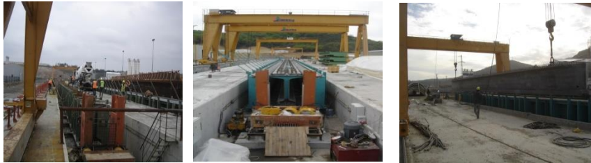
Figures 1,2, 3: Production facility of pre-stressed girders at Uskumruköy.
