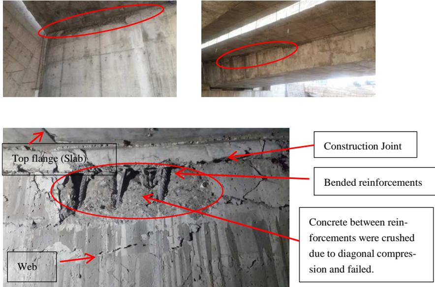
**Fig. 4.** Horizontal cracks at web-slab intersection
