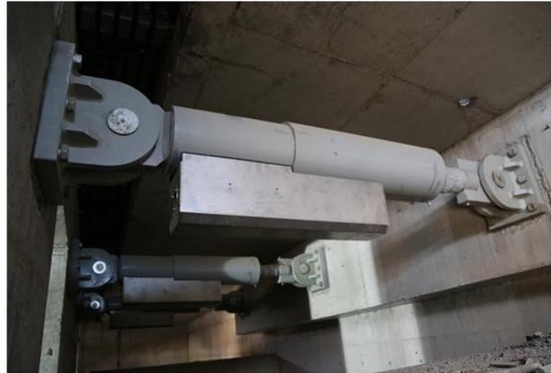
Figure 6. FVD application for bridge. Bearing definition on the piers are shown in Figure 7.
