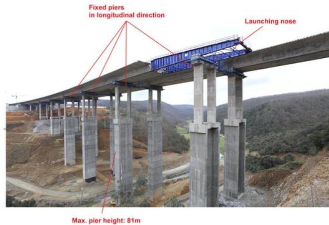
Figure 4. Viaduct V06 – Elevation view
