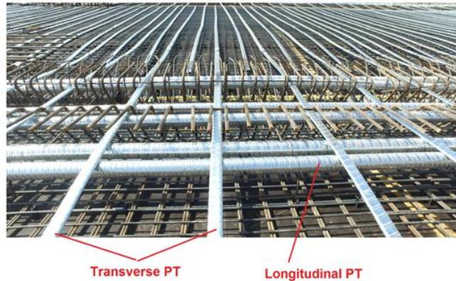
Figure 3. Transverse and longitudinal PT layout.
