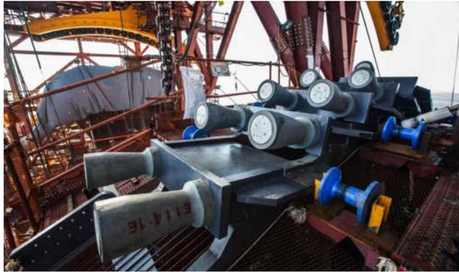
Fig. 7: Anchoring of the additional strands on a tower saddle
