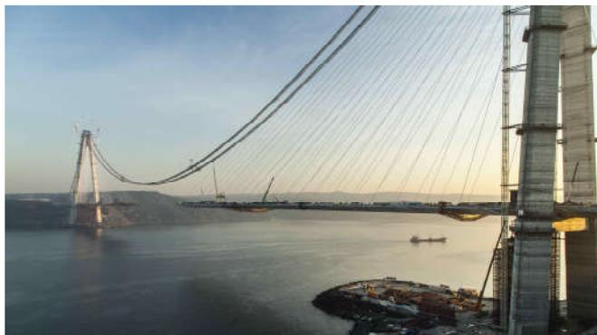
Fig. 13: Maximum cantilever erection phase
