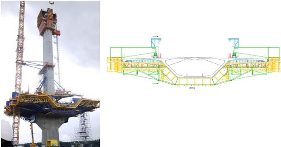
Figure 12: Mersey Cable Stayed Bridge: Flint and Neill and FHECOR: Travellers for the construction of the main spans [6]
