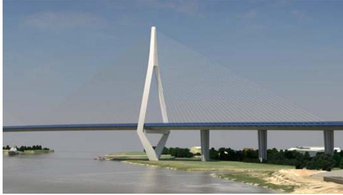
Figure 3: Single central plane with diamond shape's pylons
